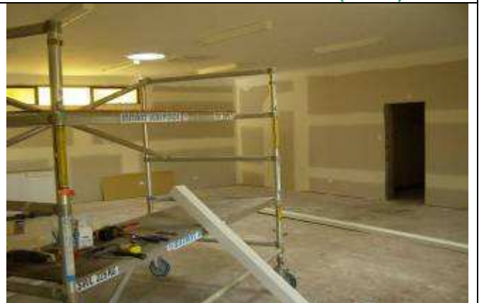
View from front of Disabled Wash Closet (SE)
