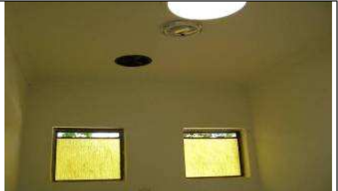
Disabled Wash Closet under construction
