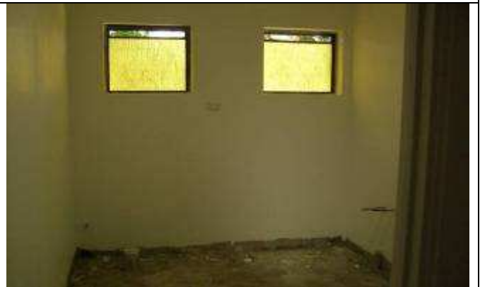
Disabled Wash Closet floor preparation
