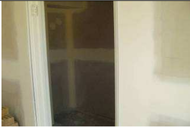
View of Store Room (rear of building)
