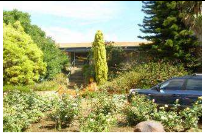
View of front of building from Office below
