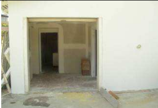
View of Entry from rear of building
