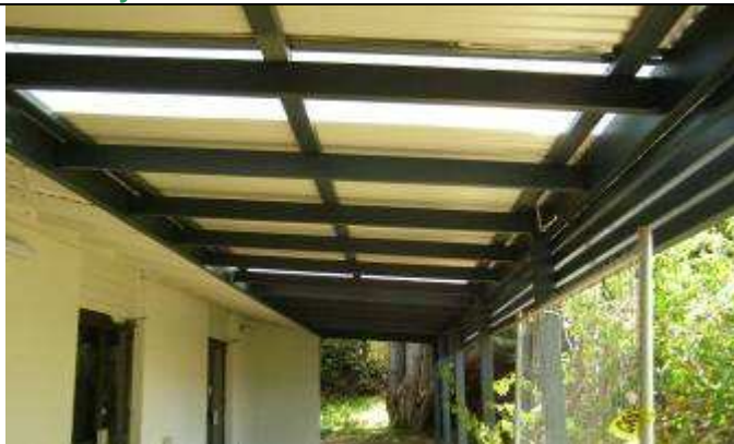
Patio Roof from South End
