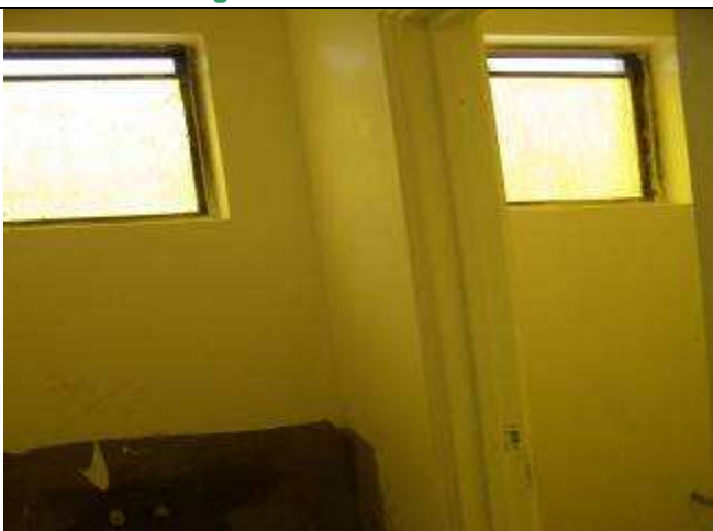
View of revamped Wash Closet
