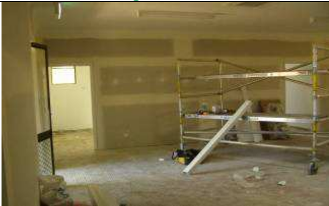
View of Training Area North End
