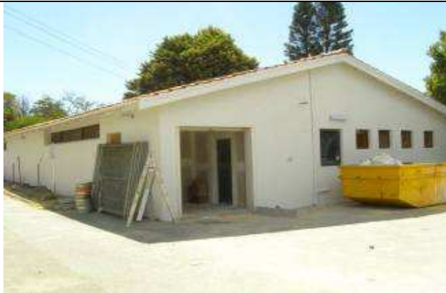
View of rear of building
