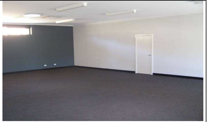
Main Room from right – door painted, skirting in.
