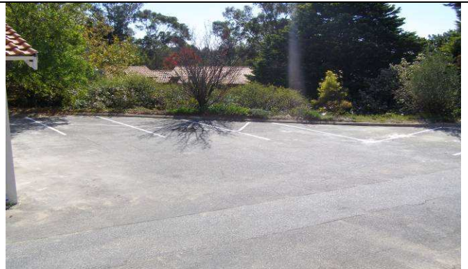
Parking bay lining completed for 5 bays.
