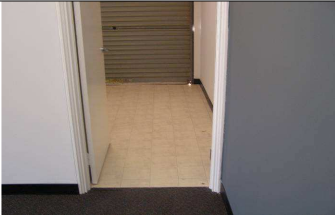
Rear store entry completed.
