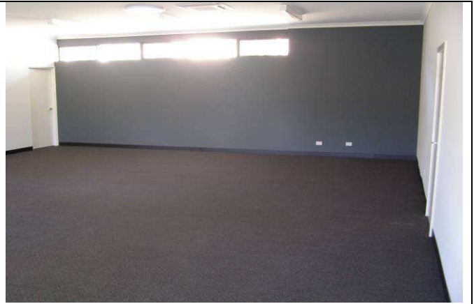
Main Room – feature wall painted, skirting done.
