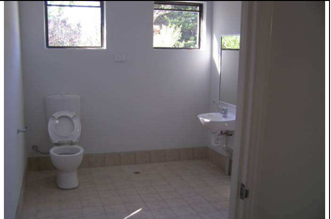
Disabled wash closet completed.
