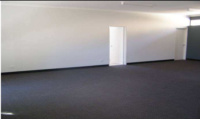
Main Room from left – doors painted, skirting done.
