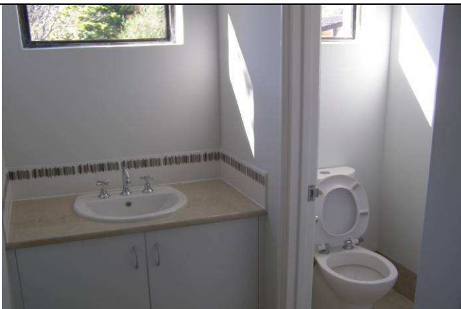
Second wash closet completed.
