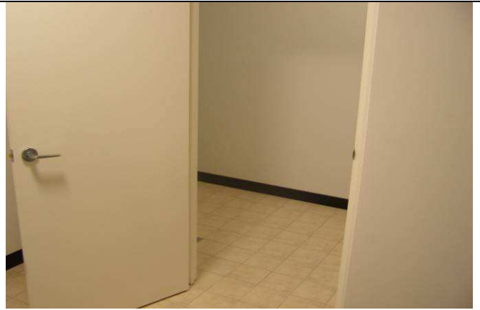
Rear store room completed.
